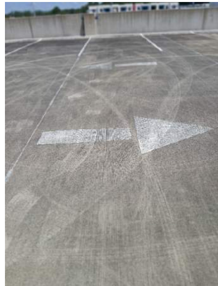
Parking Garage Top Level
