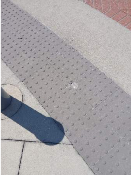
Outside Fairfield Inn & Suites
