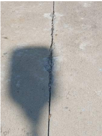
S Side of Fairfield Inn & Suites
