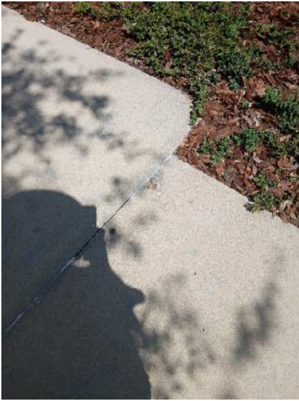
S Side of Fairfield Inn & Suites
