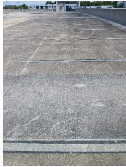
Parking Garage Top Level
