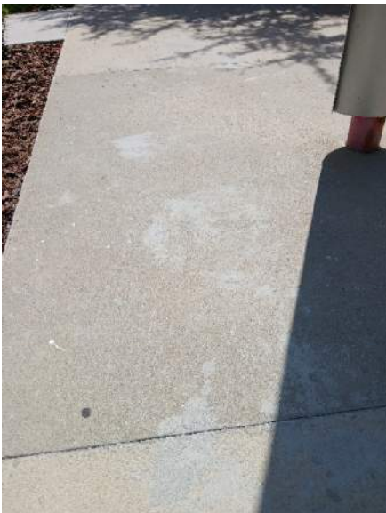
S Side of Fairfield Inn & Suites
