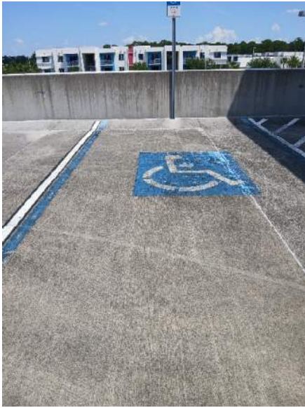
Parking Garage Top Level
