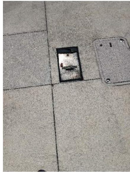
Recessed Panels in Stage Area
