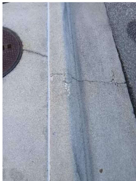
Gutter on W Side of Daytona Blvd., N of Checkered Flag Blvd.
