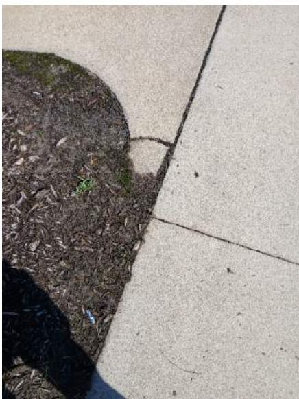
W Side of Entrance Road
