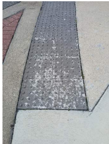
S Side of Fairfield Inn & Suites
