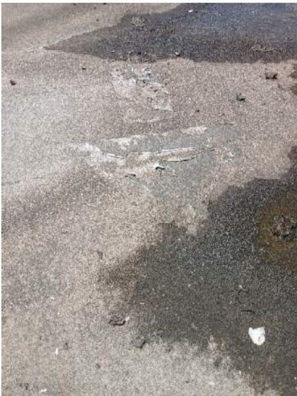
Parking Garage Top Level
