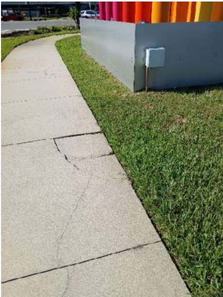
E Side of Entrance Road, Near ISB
