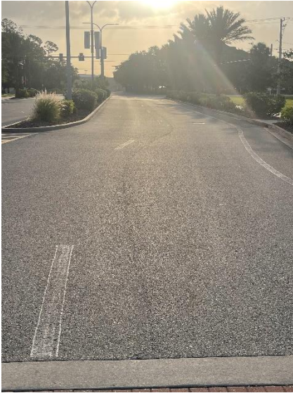
Faded Striping Location: Checkered Flag Blvd. Entrance to One Daytona Blvd. from Bill France Blvd.
